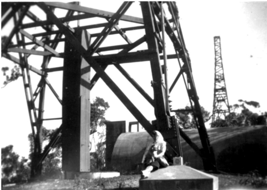
Under the Receiver Tower, 208RS
